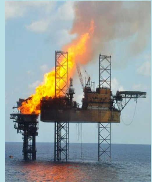
The rig on fire yesterday morning
